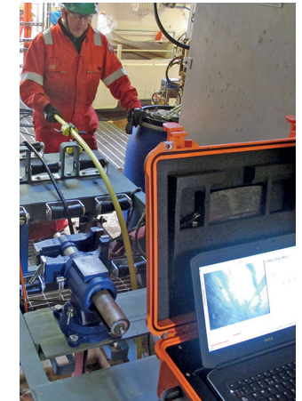
The PISCES system set up on location.
