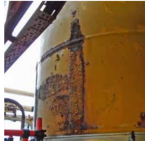
Crane pedestal before and after
